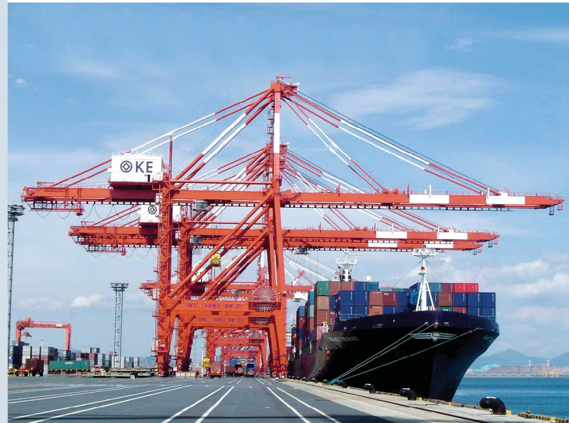
61t Quayside Container Crane
