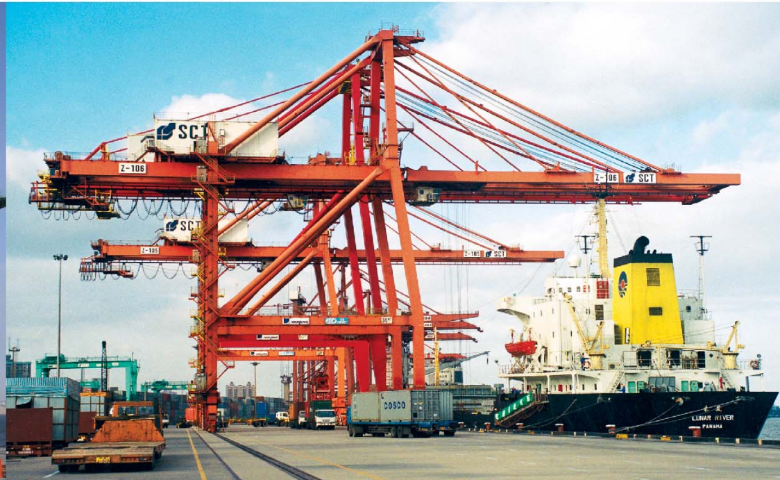
35t Quayside Container Crane in SCT Terminal, Shanghai
