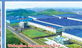
Wafangdian Manufacturing Base
