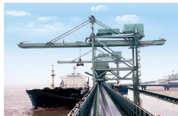
2250 t/h Ship Unloader in Shanghai
