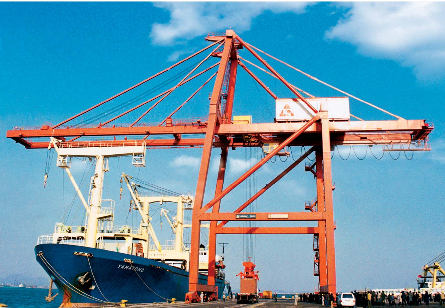
30.5t Quayside Container Crane in Dalian Port
