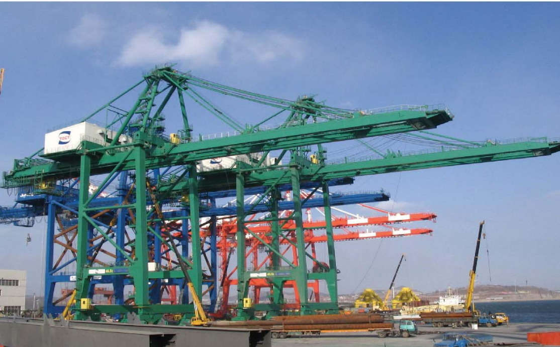
65t Quayside Container Crane in Tianjin Oriented Container Terminal
